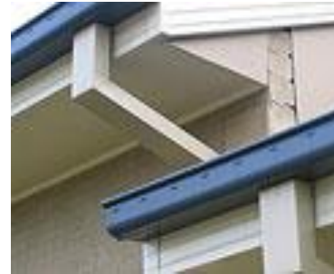
GUTTER / FACIA / DOWNPIPE
